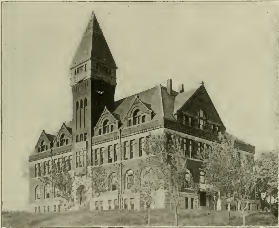
MAIN BUILDING, FAIRMOUNT COLLEGE.
