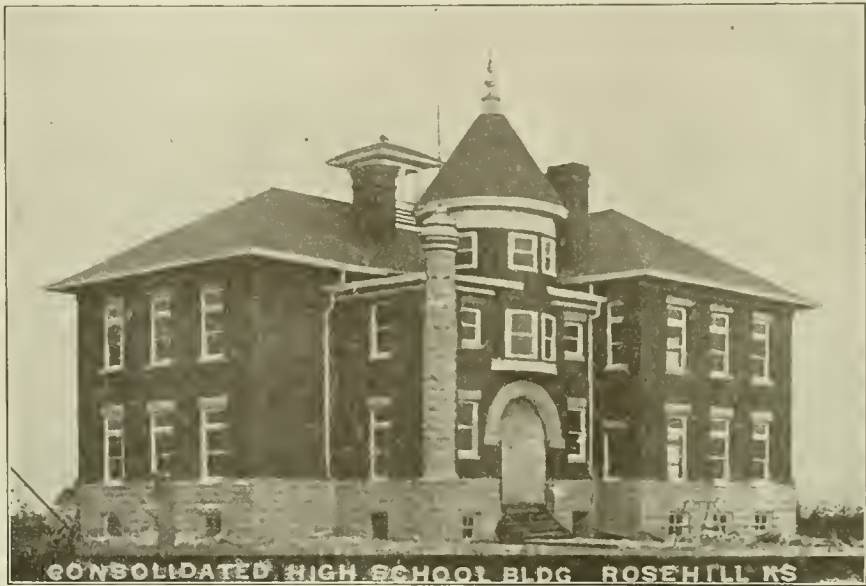
CONSOLIDATED SCHOOL AT ROSE HILL.
